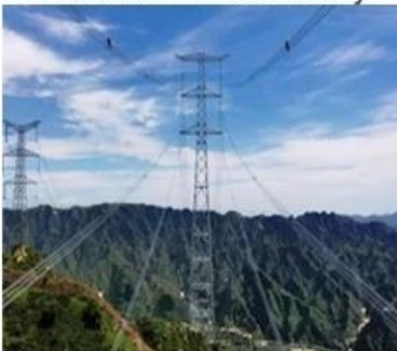
Communication base station
