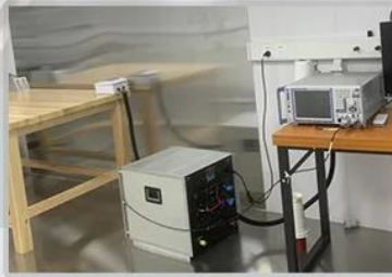
EMI Test Room
